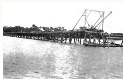
The first bridge to connect Vero Beach to the barrier island, made of palmetto logs.
