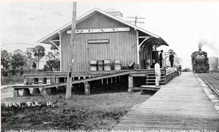
Left: Quay (now known as Winter Beach) Railroad Station was built by the Florida East Coast Railway some time between 1894-1898 of cypress and pine. It stood on the east side of the railroad tracks, south of Winter Beach Road, utilized as a produce and freight depot.
